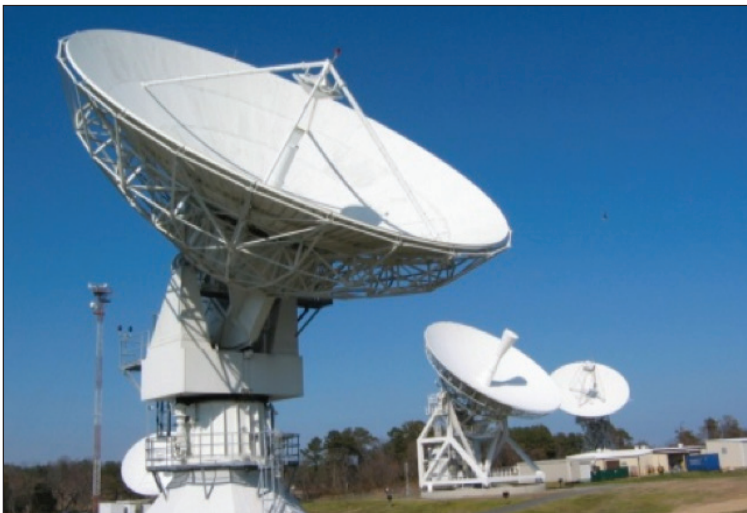
Fig. 1.4: Satellite dish for communication
