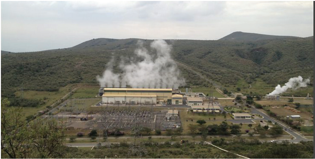
Fig. 6.8: Geothermal power station
